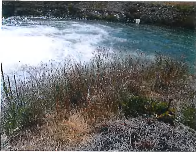
Banks of St. Mary/Milk River Diversion near Babb, MT. 10 miles from Cardston County
