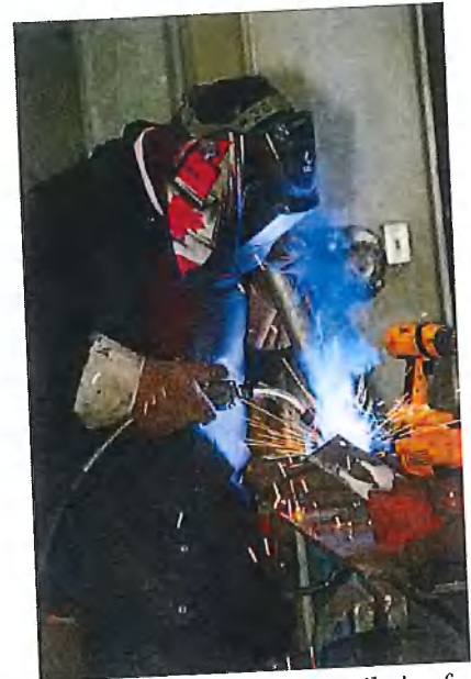
Ensure there is adequate ventilation for any indoor job where carbon monoxide is being created.
