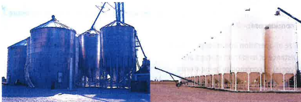
Figure 5. Steel Grain Bins (Corrugated and Smooth Walled)
