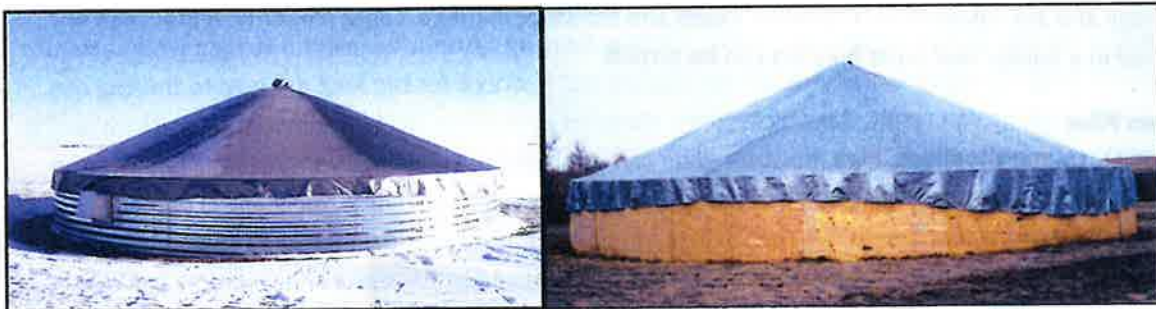
Figure 10. Grain Ring and Tarp System (Steel and Wood)
